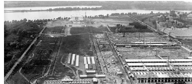
THE MAIN NAVY AND MUNITIONS BUILDING PROVIDED TEMPORARY QUARTERS FOR THE MILITARY UNTIL THE 1970S. COURTESY OF THE LIBRARY OF CONGRESS.
